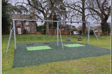
**Finding:** The seat clearance from finished surface level to the underside of the seat is too low and does not meet the requirements of BS EN 1176 Part 2 (350mm minimum clearance required)
