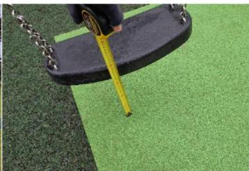
**Action:** Adjust seat height/s (400mm-500mm is recommended)
