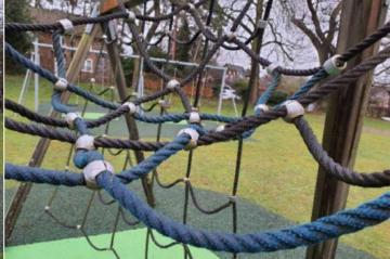
Finding: The ropes/nets are worn/damaged in places
