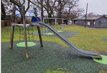
**Finding:** There is/are finger entrapment/s in the slide starting section and the item fails to meet the requirements of BS EN 1176 Part 1 4.2.7.6 Entrapment of fingers
