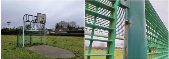
Finding: The paintwork on this item has been damaged or Action: Treat affected areas and repaint worn exposing the metal underneath which is rusting / corroding
