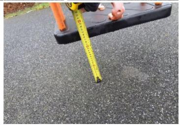
**Finding:** The seat clearance from finished surface level to the underside of the seat is too low and does not meet the requirements of BS EN 1176 Part 2 (350mm minimum clearance required / currently 220mm)
