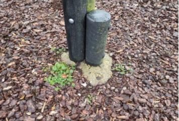
**Finding:** The exposed foundation forms a hard object within **Action:** Top up loosefill levels to cover foundations the impact area of the equipment in contravention of the requirements of BS EN 1176 Part 1
