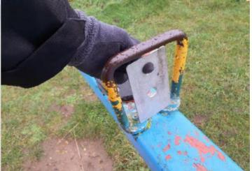
Finding: The item fails to meet the requirements of BS EN Action: Monitor - No remedial work recommended 1176 Part 1 4.2.7.2 for head and neck entrapment in the frame
