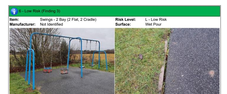
**Finding:** There are gaps opening between the surfacing and **Action:** Monitor for any further deterioration and repair as the edging surround or between the joints in the surfacing required
