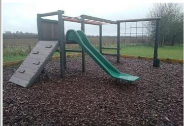
**Finding:** The timber edge forms a hard object within the falling space of the equipment in contravention of the requirements of BS EN 1176 Part 1
