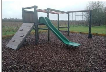
Finding: The ropes/nets are worn/damaged in places
