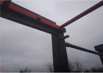
Action: Replace missing inserts to remove entrapment
