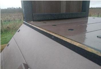
Action: Replace the damaged edging strip
