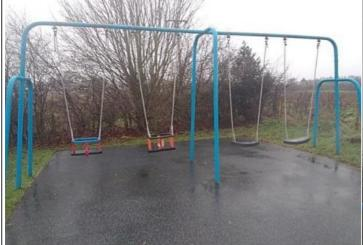
Action: Cut back excessive chain links Finding: There are excessive chain tails
