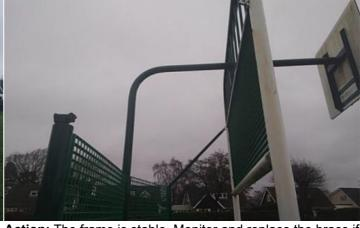
Finding: A support brace has been removed/not fitted
