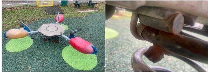
Finding: The paintwork on the spring has been damaged or Action: Treat any rusting components and repaint worn exposing the metal underneath which is rusting
