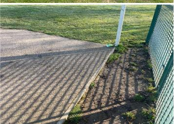
Finding: There are trip hazards at the edges of the surface Action: Reinstate surrounding surface levels to remove the
