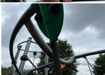
Finding: The ropes/nets are worn/damaged in places
