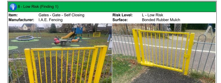
**Finding:** The gate is closing too quickly (less than 4 seconds)
