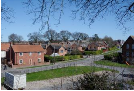
Recent development, Station Hill
